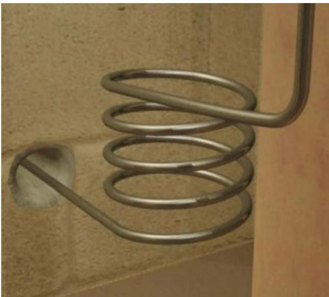
Expansion coils exiting the furnace
